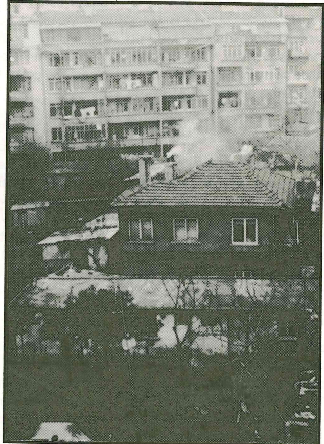
Overcrowded cities with massive transport and housing problems
